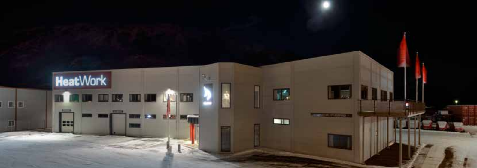
HeatWork headquarter and production site in Narvik, Norway – 3300 m 2 state of the art production facilities.
